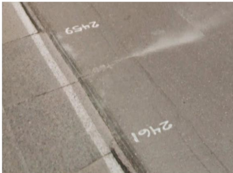
a) Cell 61: FSR_{\text{Winter}}=0.9 , PCC = 127 mm (5 in), Asphalt = 178 mm (7 in)
