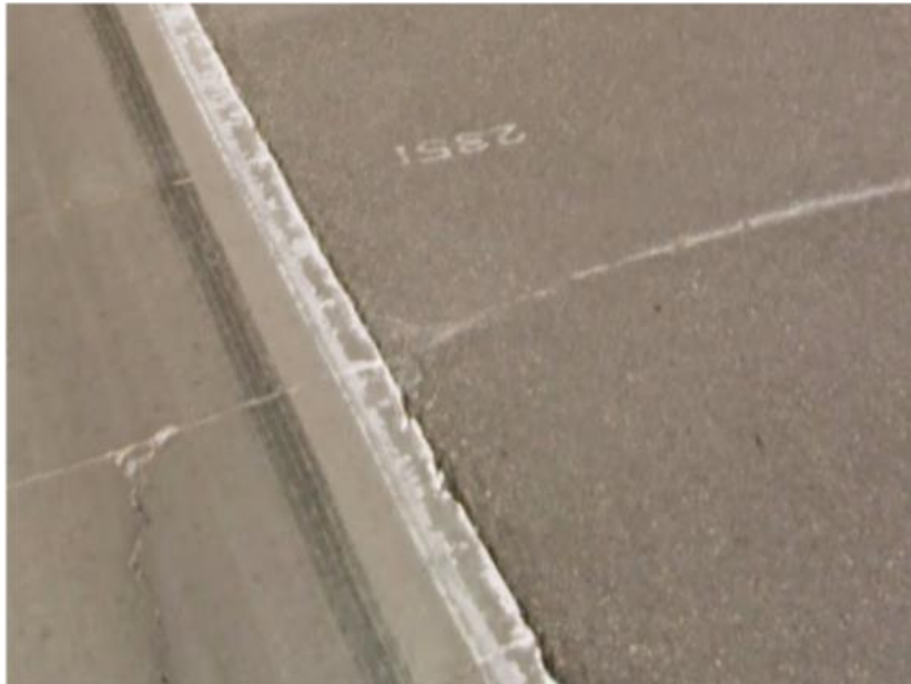
a) Cell 61: FSR_{\text{Winter}}=0.9 , PCC = 127 mm (5 in), Asphalt = 178 mm (7 in)
