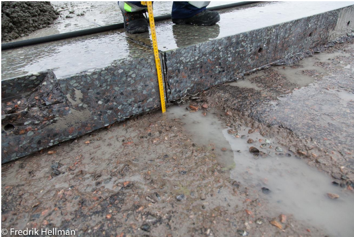
Figure 6 – Erosion of the cement treated base visible under a removed, cracked slab.
