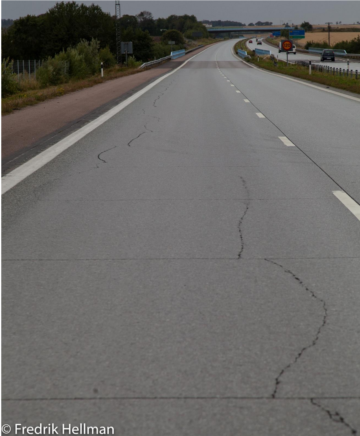
Figure 4 – Longitudinal cracking in wheel track (photo taken against traffic direction).
