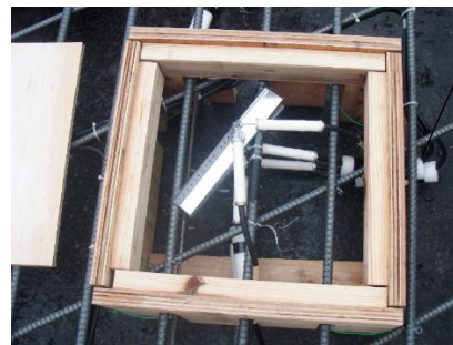
Figure 5. Sensor Installation at a Measurement Point.
