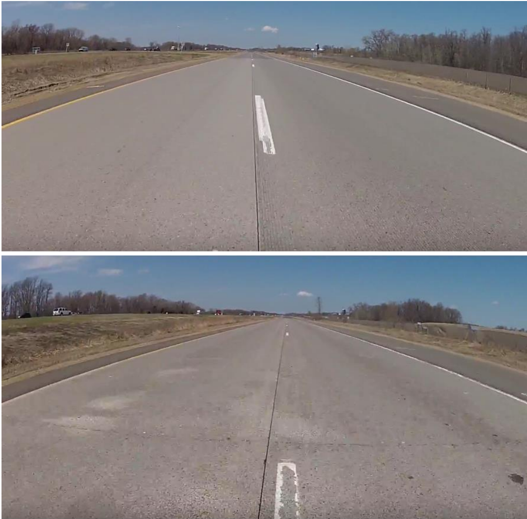
Figure 2. MnROAD Cell 71 (top) and Cell 72 (bottom) as of November 2013
