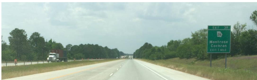
Figure 1-Showing new outside lane and new RCA PCC shoulders
