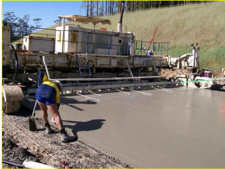
Figure 4. 10m wide slipform paving of LMC subbase with steel float finish
