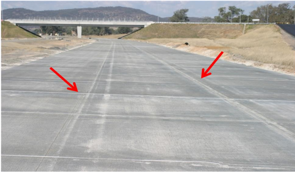
Figure 17 . Full width highway PCP construction with sawn longitudinal joints (see also Fig15) shown. Prior to lane marking.
