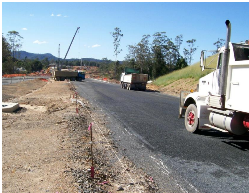
Figure 12. Trucks hauling subbase LMC on sealed SMZ
