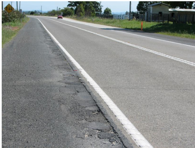
Figure 9. Concrete pavement without concrete shoulder
