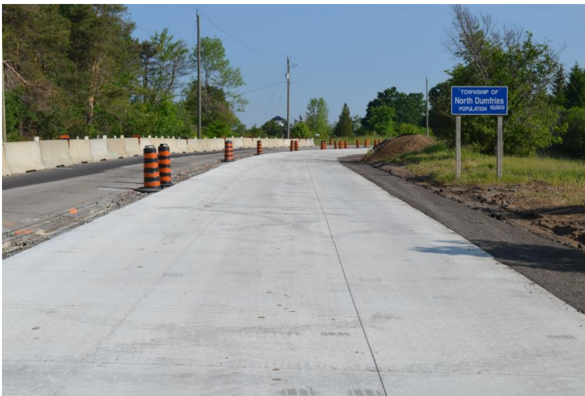
Figure 7: Northbound concrete pavement with RAP shoulder (Priour 2015).
