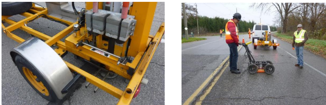
Figure 3: FWD and GPR Investigations Photos (Holt 2014).
