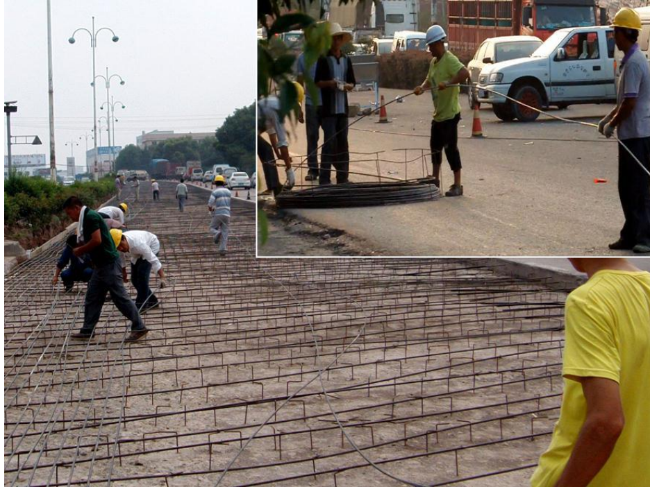
Figure 2. Placement of longitudinal BFRP on transverse chairs.
