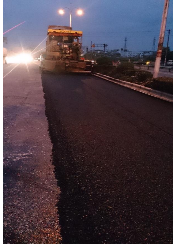
Figure 7. Construction of the asphalt overlay.
