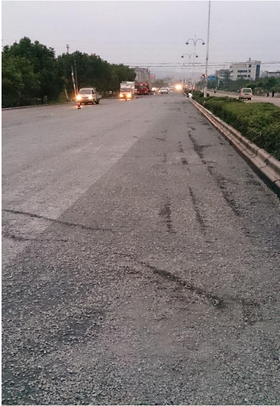
Figure 6. Construction of the SMA interlayer.
