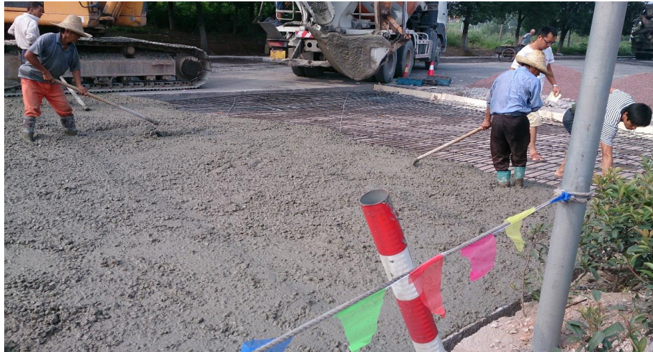
Figure 4. Concrete casting for CRCP with BFRP bars.
