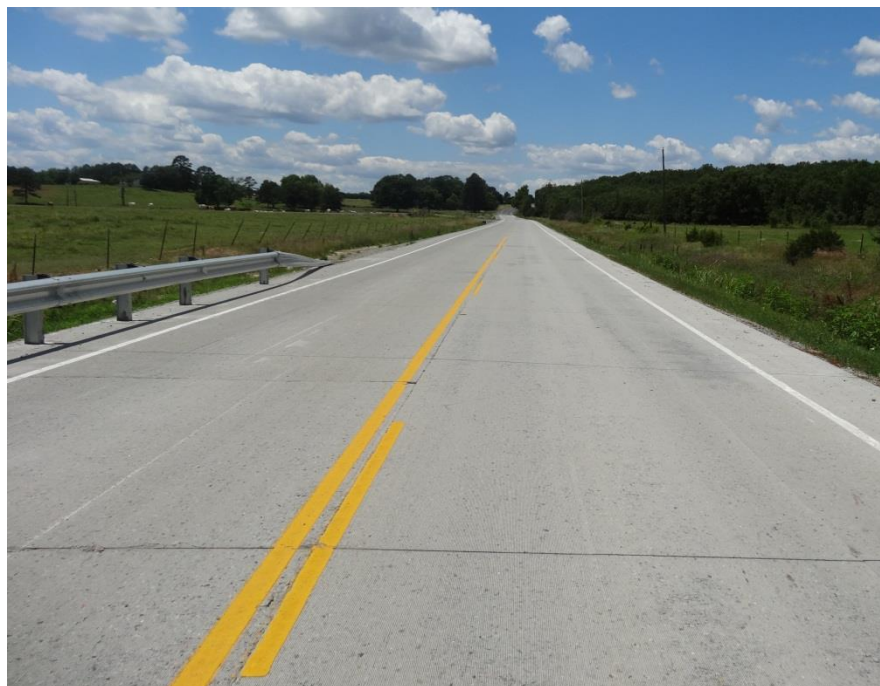
Figure 1. Arkansas Highway 213 RCC Pavement Project
