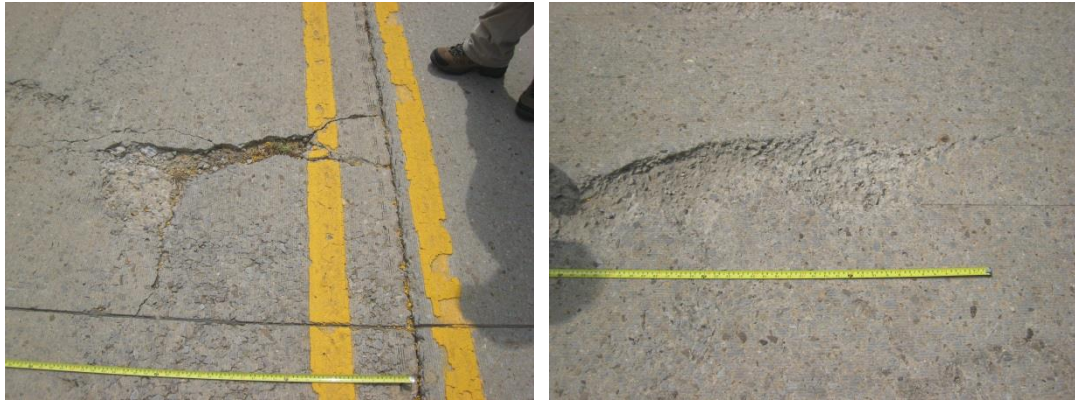
Figure 8. Examples of raveling.
