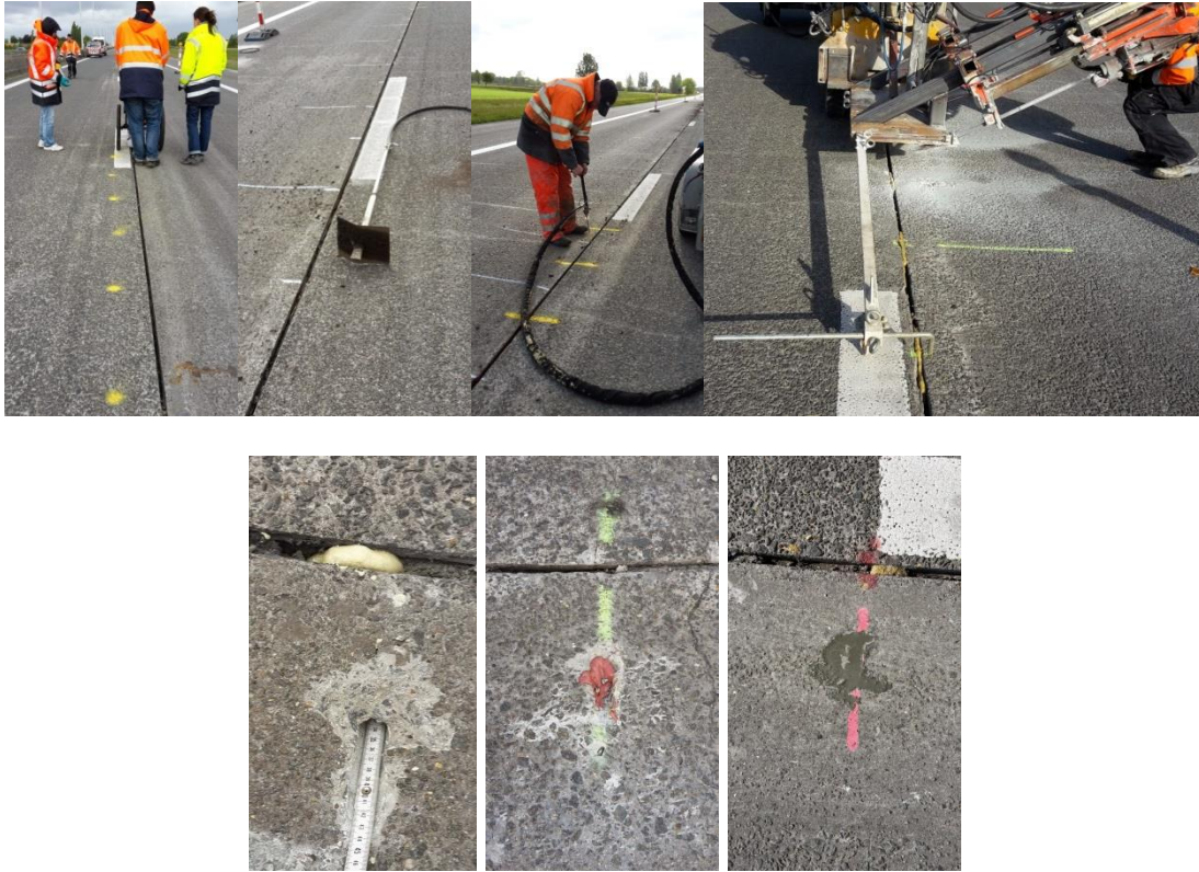
Figure 9. Different steps of stitching: positioning of the existing tie bars; cleaning of the joint (and damming); drying of the joint; filling up the joint with polyurethane foam (no picture); drilling the holes (two at the time); insertion of the tie bars in the epoxy glue; filling up the surface with acrylic resin.
