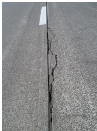
Figure 2. Widening of the longitudinal joint and cracking over a width of 100 to 150 mm along the joint
