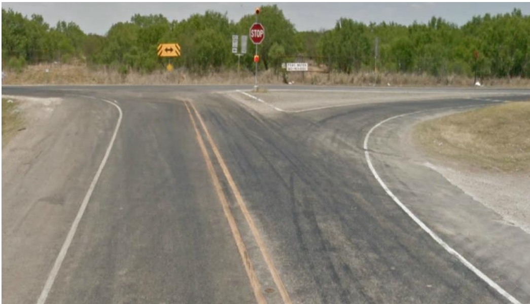
Figure 4. TxDOT PCP project – view west on SH 72 at intersection with SH 97.
