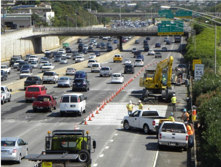
Figure 3. PCP inlay utilized by HDOT across five lanes of H-1.
