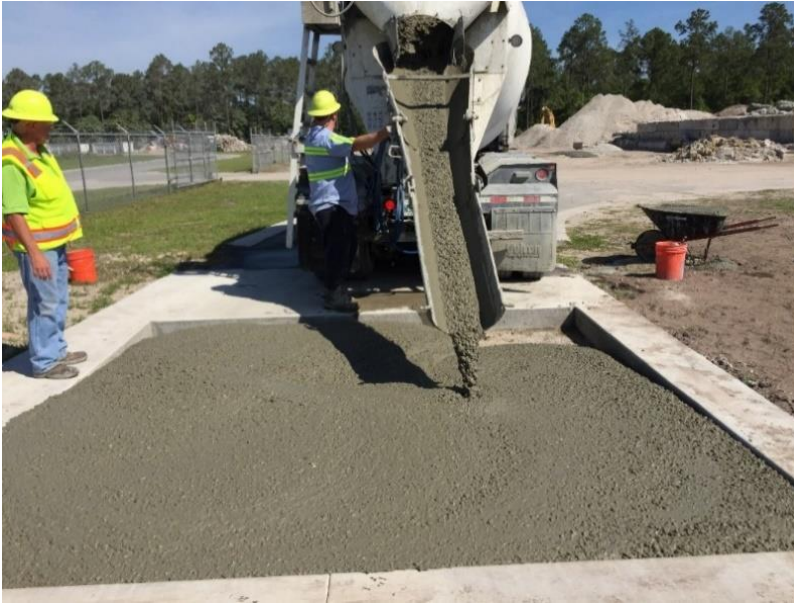
Figure 7. Casting SCC mix in replacement slab pit at test track
