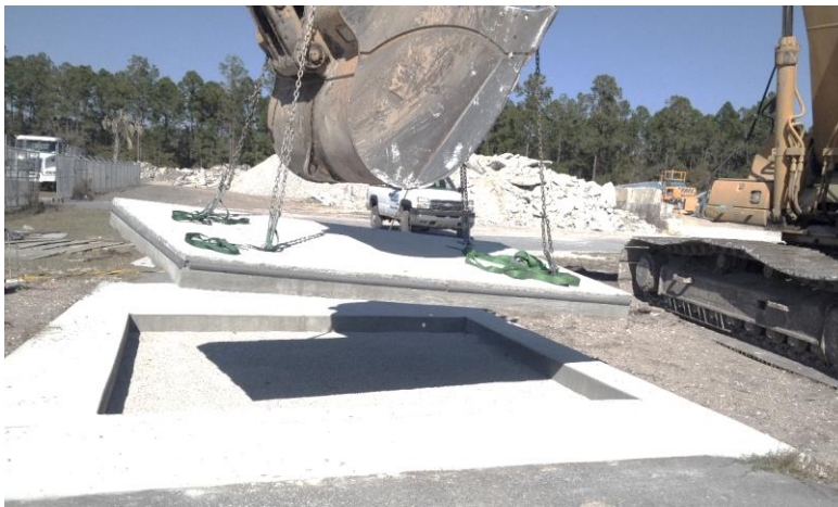
Figure 5. Rigged precast panel for installation in slab replacement pit
