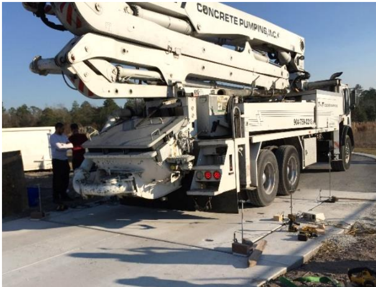
Figure 6. Load testing of precast panels
