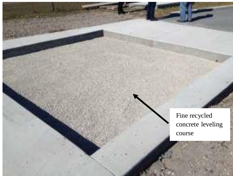
Figure 3. Test pit with fine recycled concrete aggregate leveling course
