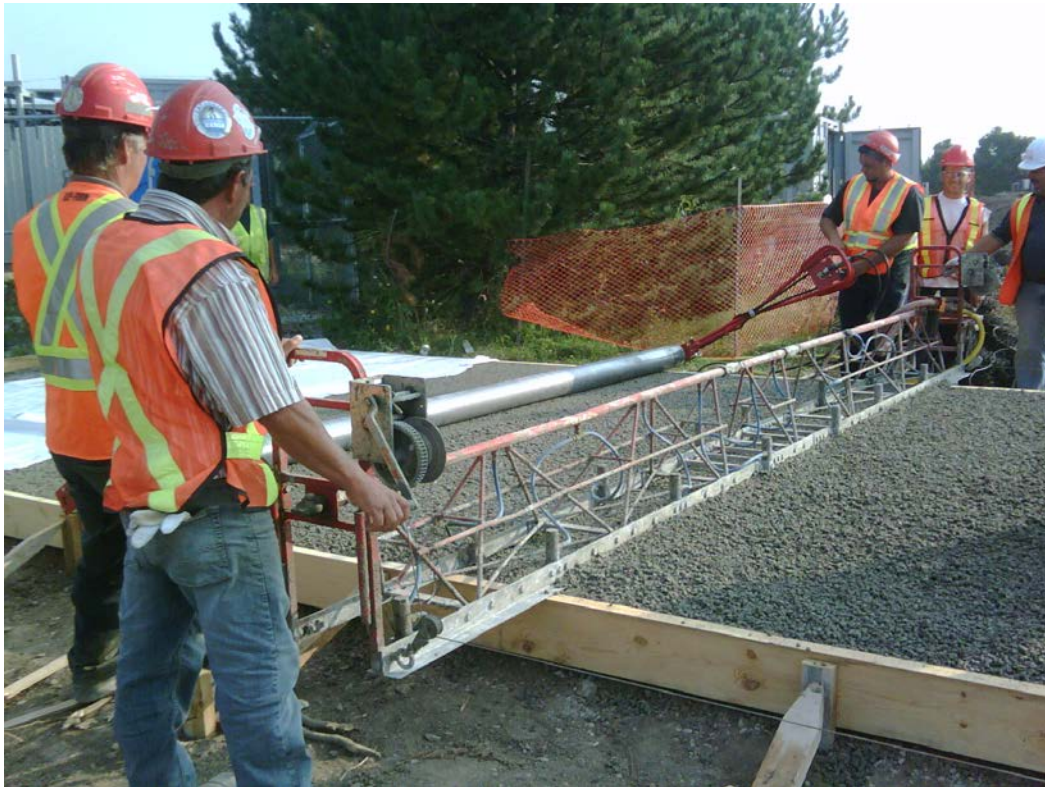
Figure 2. Trial Vibratory Screed on 10 mm strips followed by Hydraulic Roller
