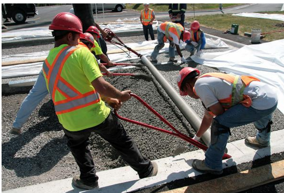
Figure 3. Hydraulic roller screed running along pervious concrete and curb & gutter
