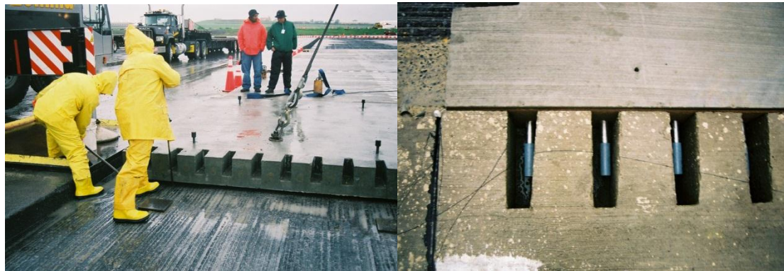
Fig. 6. Alternate Scheme for Providing Load Transfer in JPrCP (Tayabji, Ye, Buch, 2011).
