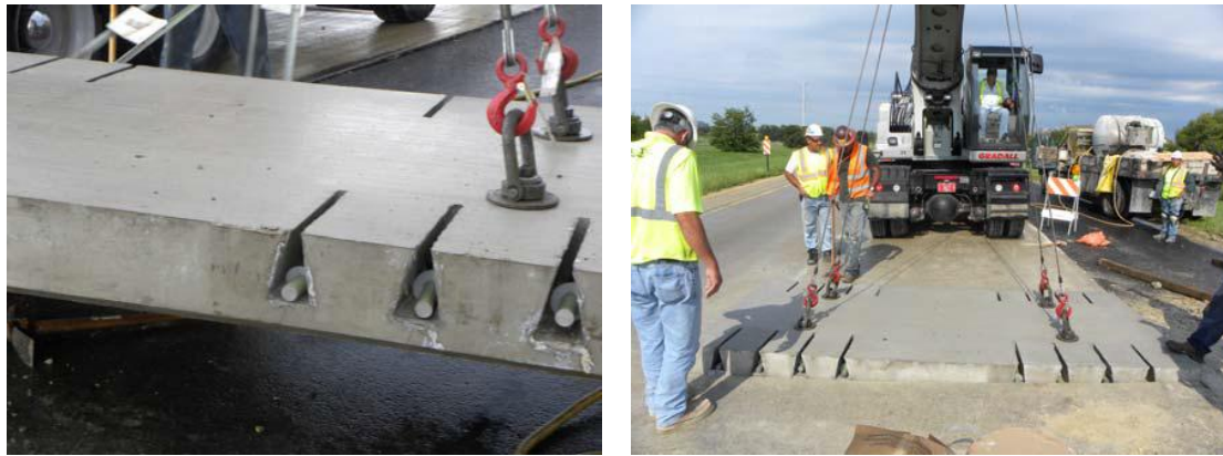
Fig. 9. Narrow-mouth surface dowel slots (Tayabji, Ye, Buch, 2011).
