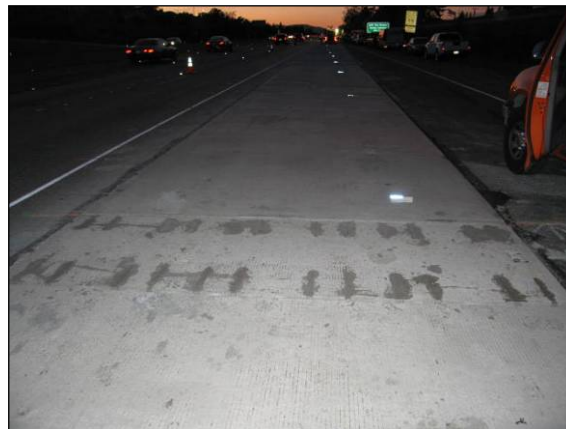
Figure 13. Completed PPCP section prior to grinding.
