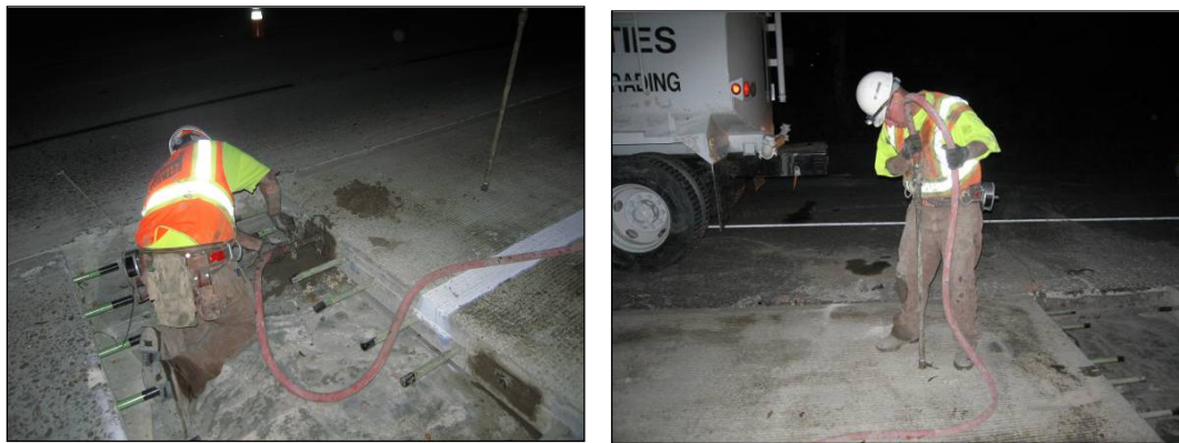
Figure 11. PT duct and underslab grouting.
