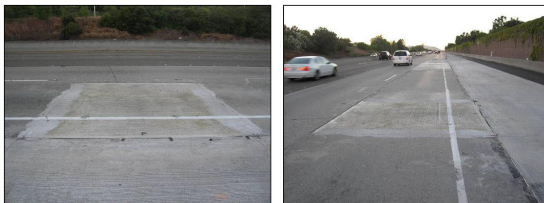
Figure 14. Completed JPPCP panels.
