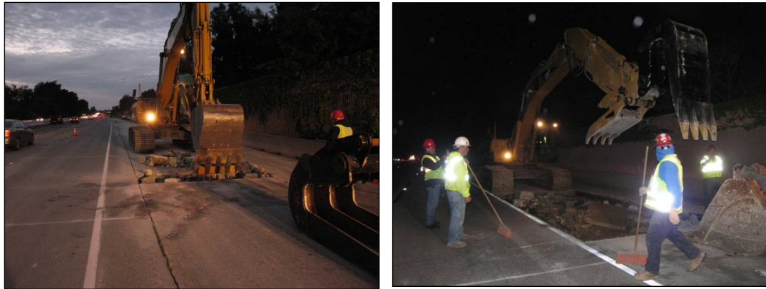
Figure 5. Removal of distressed pavement and underlying base.
