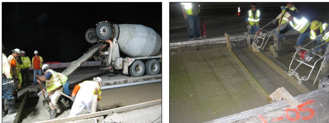
Figure 8. Placing and grading LCB-RS
