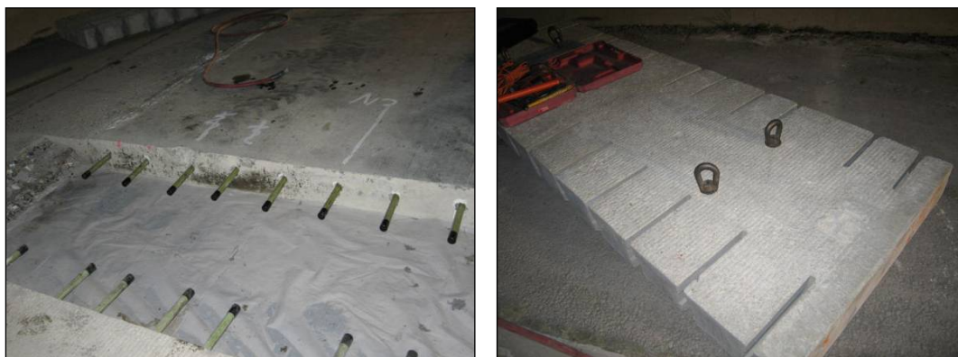
Figure 12. Dowels installed in existing pavement (left); permanent drop-in panel (right).
