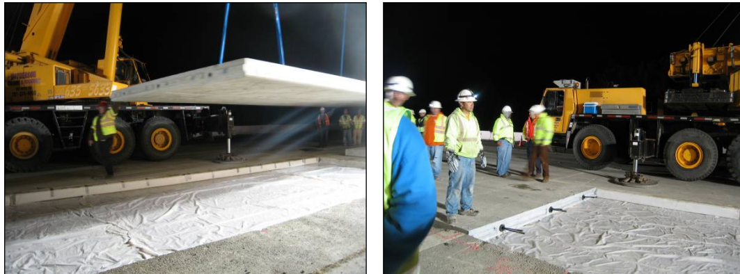
Figure 9. Installation of PPCP panels over LCB and friction-reducing membrane
