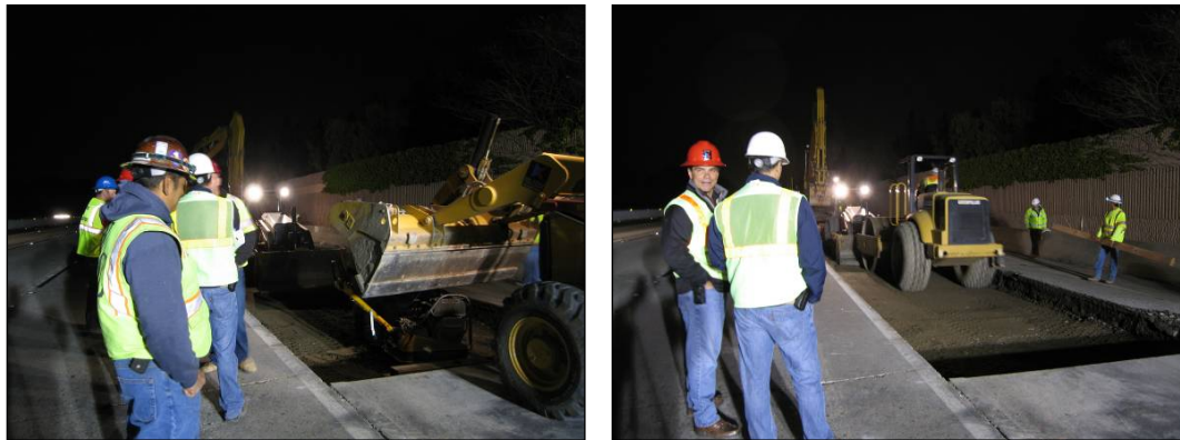
Figure 6. Grading and compaction of subbase
