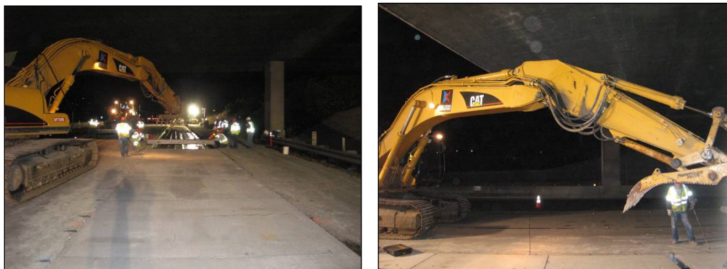
Figure 15. PPCP installation under a structure (17' clearance)
