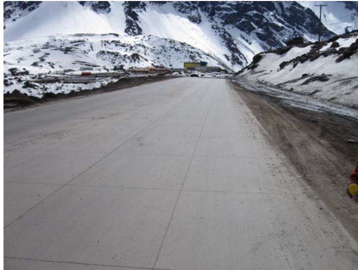
Figure 9. 15 cm FRC TCP design (2 m x 1.75 slab size) in Route 60 for 20.000.000 ESALs (2 year)
