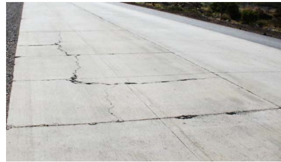
Figure 7. Slabs cracked in less than a week Figure 8. TCP design after 8 months with AASHTO design 4 m long slabs with 2 m long slabs
