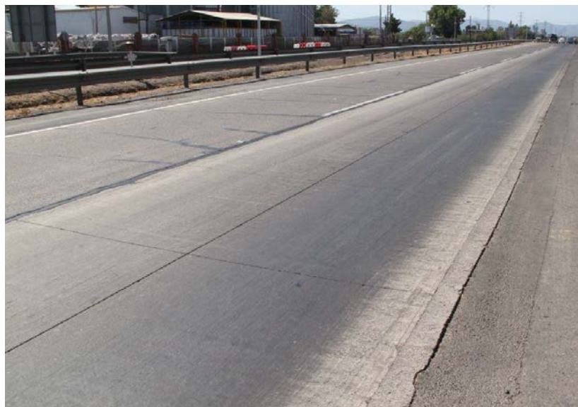
Figure 11. Route 5, 16 cm Thick with TCP design for 50.000.000 ESALs (2,5 years)
