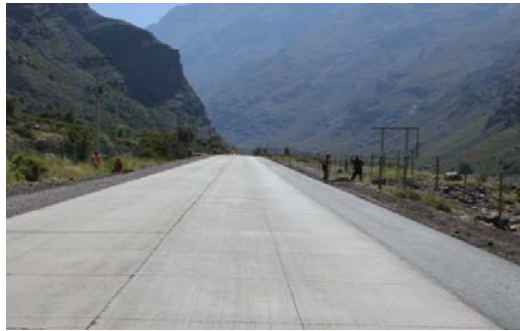
Figure 7. Slabs cracked in less than a week Figure 8. TCP design after 8 months with AASHTO design 4 m long slabs with 2 m long slabs
