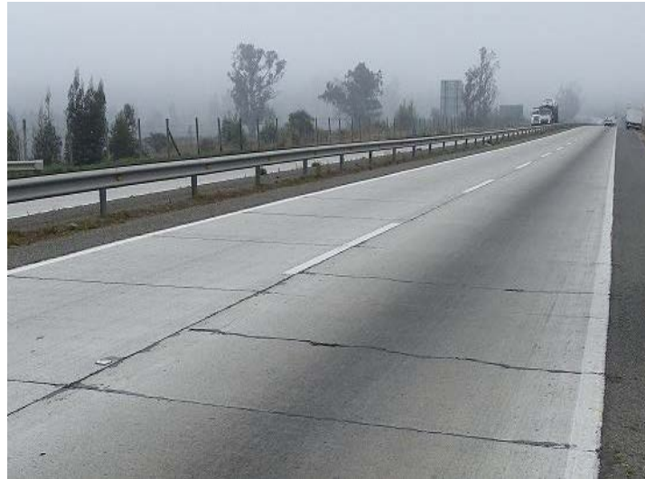
Figure 1. Route 78 Section D (Km 90.000 to Km 92.930) paved during daytime.
