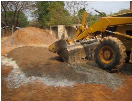
Figure 5c: Mixing RCC materials
