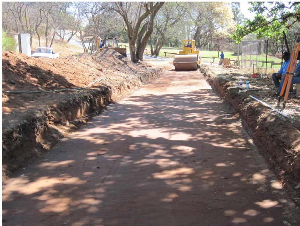
Figure 3: Subgrade preparation and compaction
