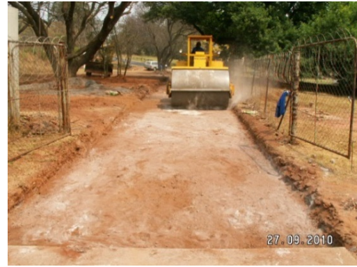
Figure 5b: Compacting base with roller-compactor
