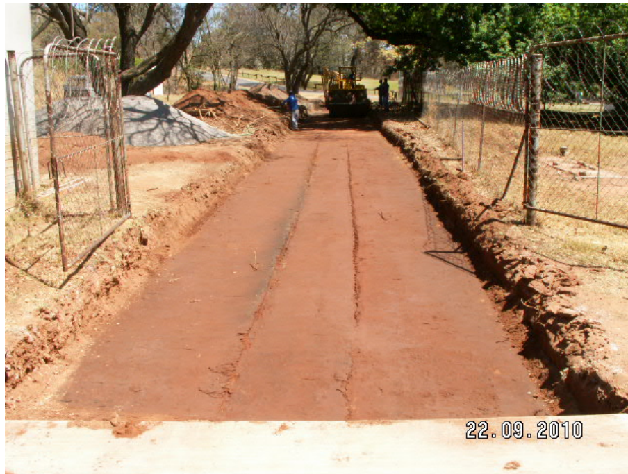
Figure 4: Subbase construction
