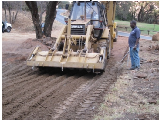
Figure 5d: Distribution of RCC materials
