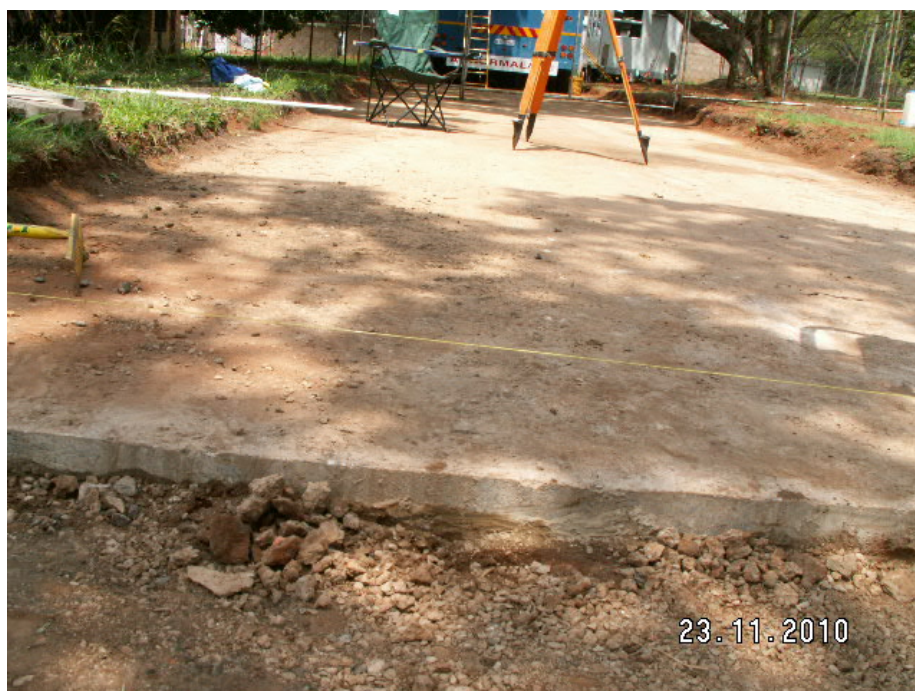
Figure 5e: RCC layer after construction of phase I (mechanical equipment)
