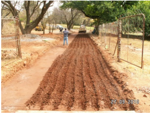
Figure 5a: Mixing cement and fly ash with in situ material
