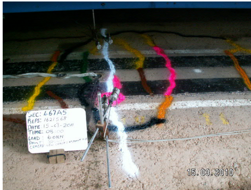
Figure 12: Circular crack pattern after 1.6 million repetitions
