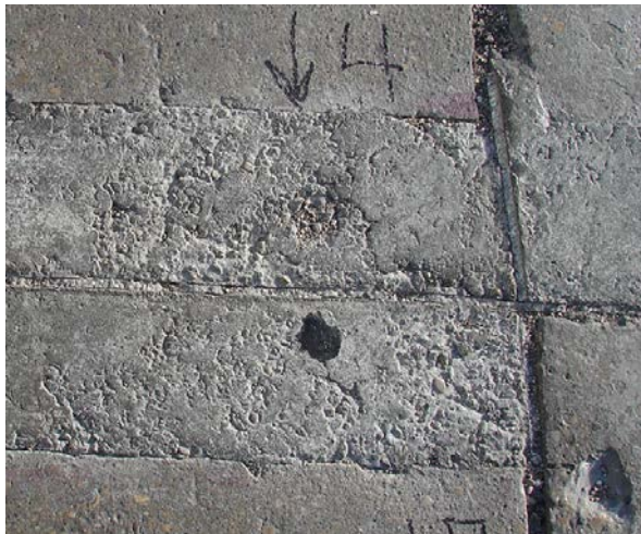
Figure 7: Repair Areas with Poor Surface Finish
