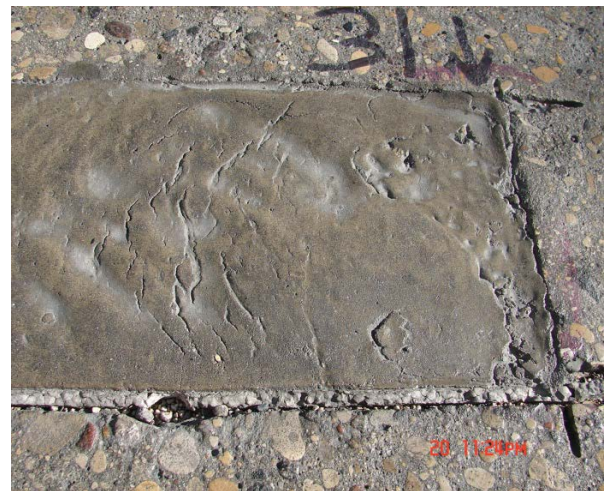
Figure 7: Repair Areas with Poor Surface Finish
