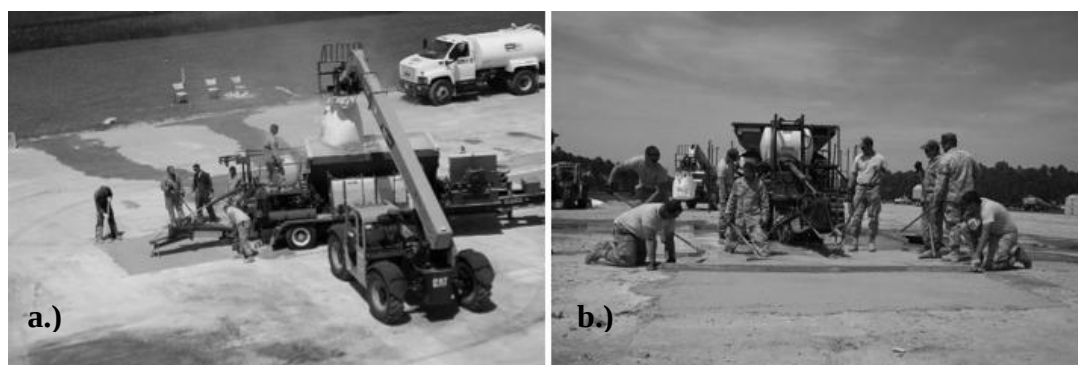
Figure 3: Capping Procedure using RS Material: a.) dispense material into excavation after observing required backfill curing period, b.) level surface using straight edge and finish using minimal handwork. Delay application of traffic until completion of manufacturer specified curing period.
