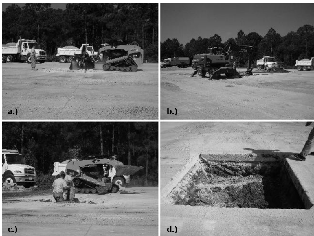
Figure 2: Excavation Preparation Procedure: a.) saw cut damaged pavement and upheaval, b.) remove damaged pavement and excavate until sound subgrade is reached, c.) trim excavation using hand tools to ensure vertical walls and level floor, d.) clear debris from surrounding pavement prior to backfill operations.
