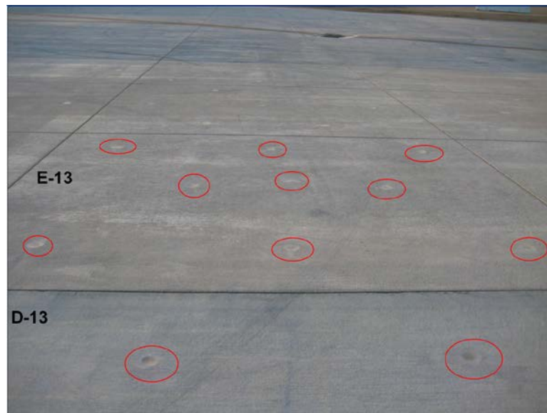
Figure 4. Slabs after being grouted.
