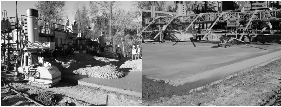
Figure 9: Two-lift photocatalytic concrete paving, in Chesterfield, MO (October 2011)
