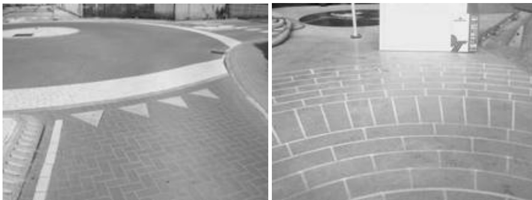
Figure 4: Two examples of paving blocks (left) and slabs (rights) applications.
