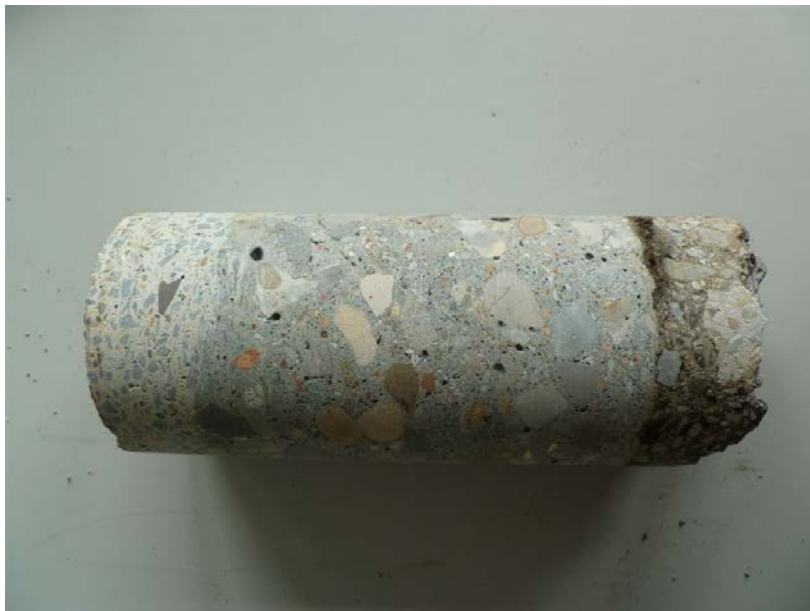
Figure 9 – Core taken from the pavement.
