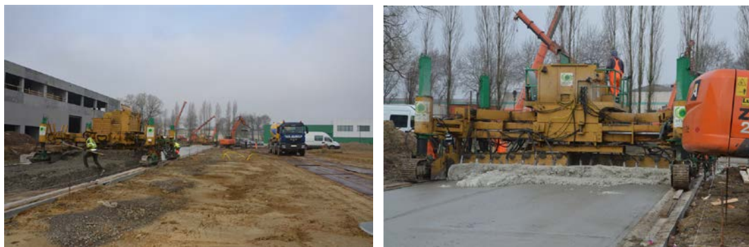
Figure 7 – Construction of the double layered concrete pavement.
