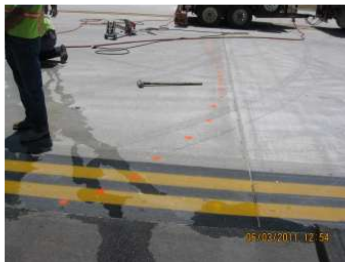
Figure 1 Hammer for Sounding Delaminated Areas (see red dots).
