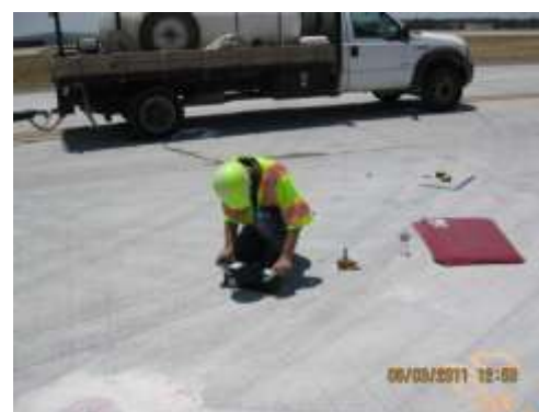
Figure 8b Using Ultrasonic Tomography in the Field.
