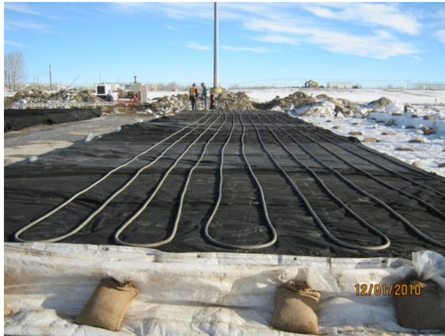
Photo 2. Installation of glycol heating lines on the PCCP.
