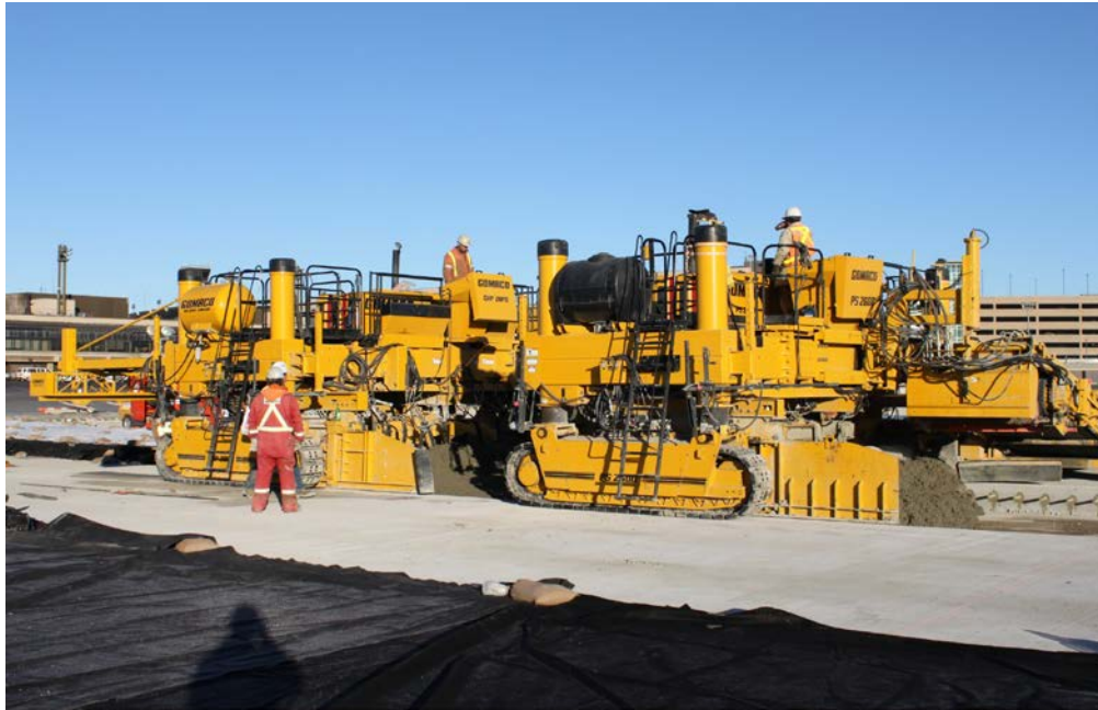
Photo 1. Gomaco's placer/spreader and paver.
