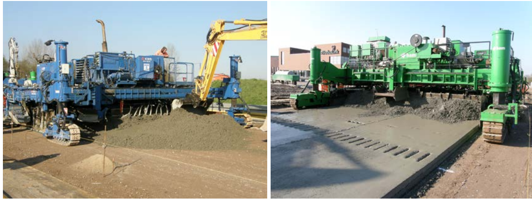
Figure 2 – Applying the bottom layer (left panel) and the top layer (right panel)
