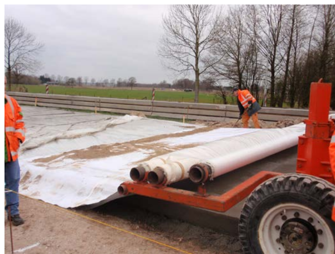
Figure 3 – Applying plastic sheet
