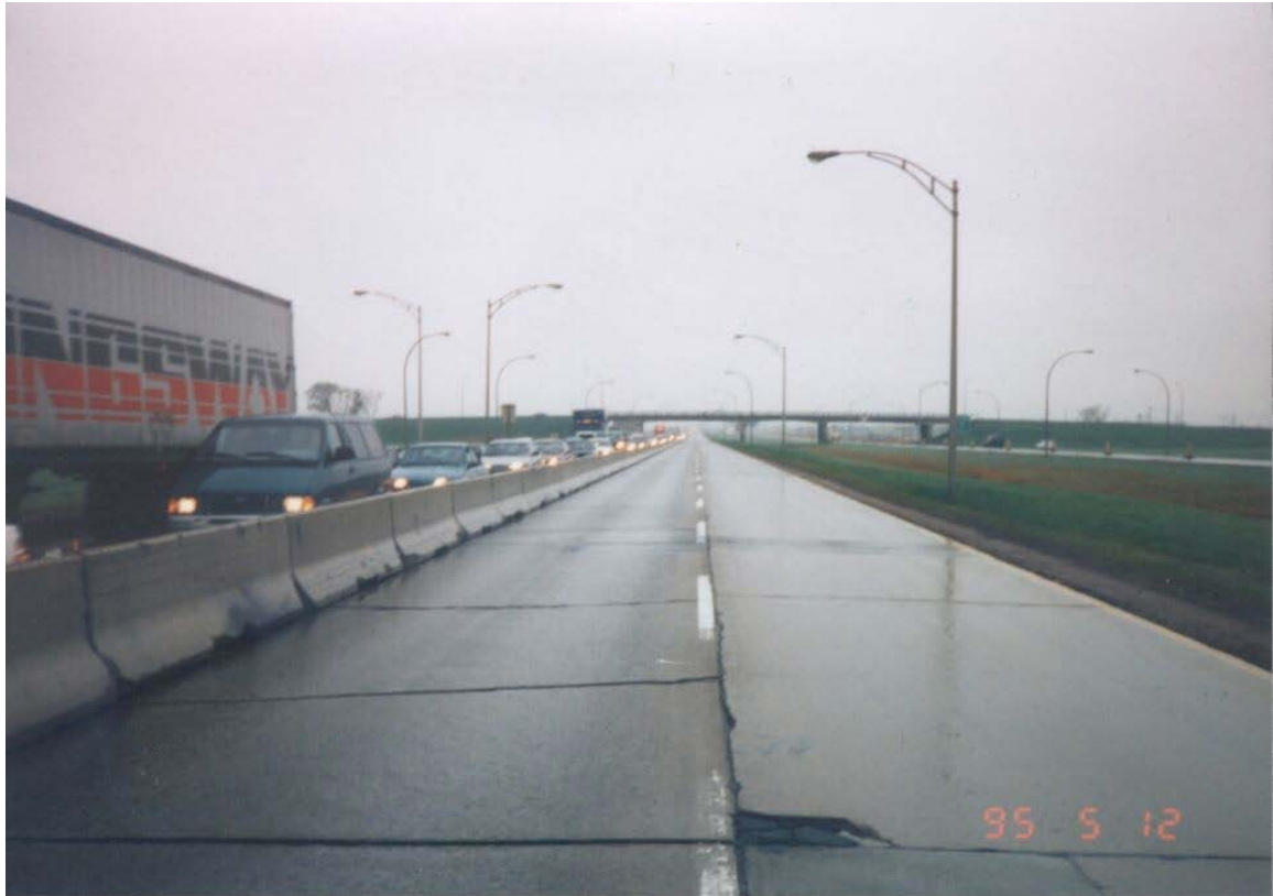
Figure 2 – Deteriorated Pavement
