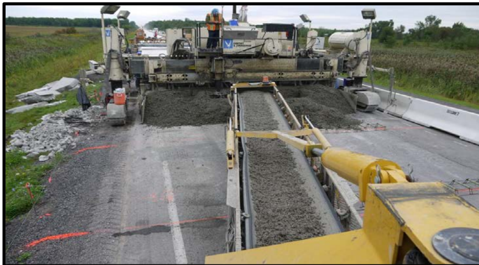
Figure 9 – Concrete Distribution in Front of the Paver
