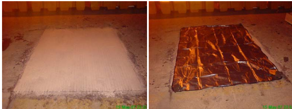
Photo 10: Repaired with rapid hardening concrete (left)
