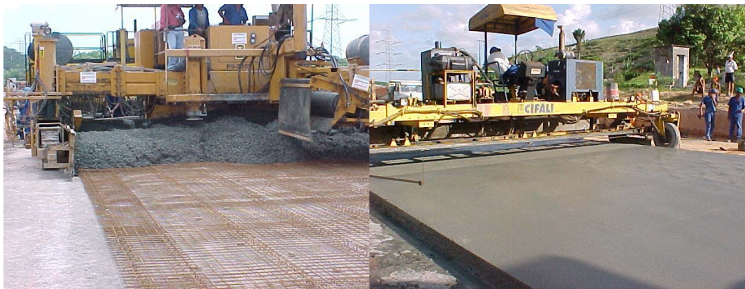
Figure 1. Using of slip-form paver for laying concrete over steel welded mesh (construction site managed by the authors; pictures by Ganassali).
