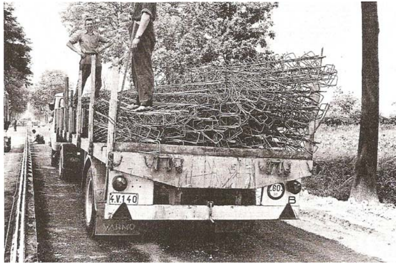
Transporting cross-reinforcements
