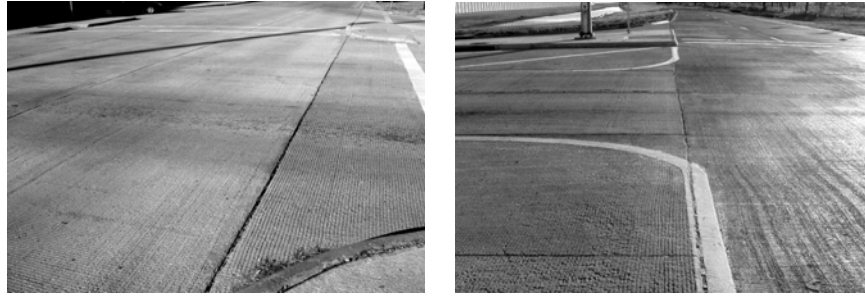
3-c) Good Performance with Proper Construction Joint between the Frontage and Cross Roads
