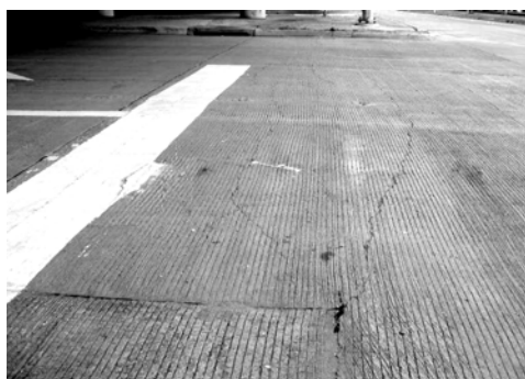
6-a) Restraint Cracking from Drainage Inlet Box
