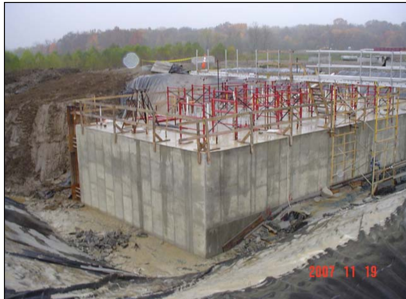
Figure 8 Concrete filled test shell
