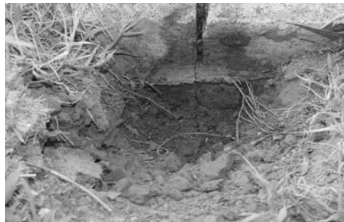
Figure 8. Verification of the development of the controlled crack across the narrow transverse contraction joints
