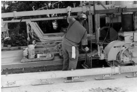
Placement of tie bars to the finished concrete pavement
