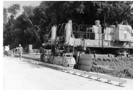
Slip form paver during pavement construction
