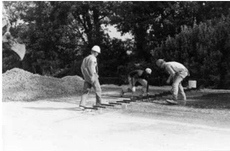
Placement of dowel bars
