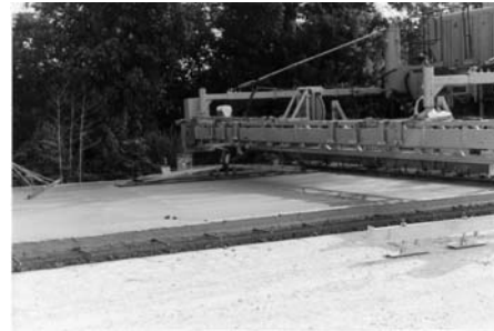
Creating pavement surface texture
