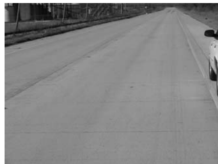
The new jointed plain concrete pavement
