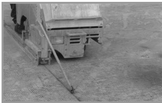
The early entry dry cutting of the narrow joints at test section S2
