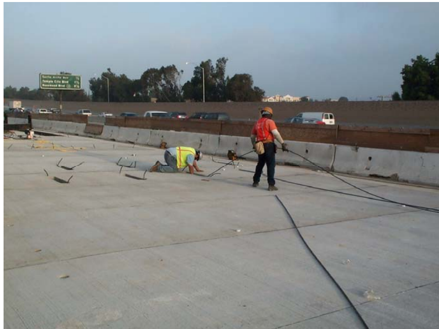
Figure 11. Workers fed the post-tensioning strands into the ducts at the pockets in the central stressing panels.
