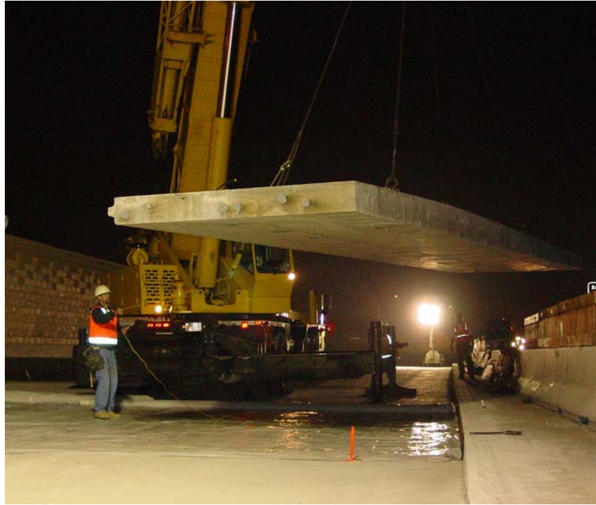
Figure 9. Each panel was lifted over the concrete barrier and set in place.
