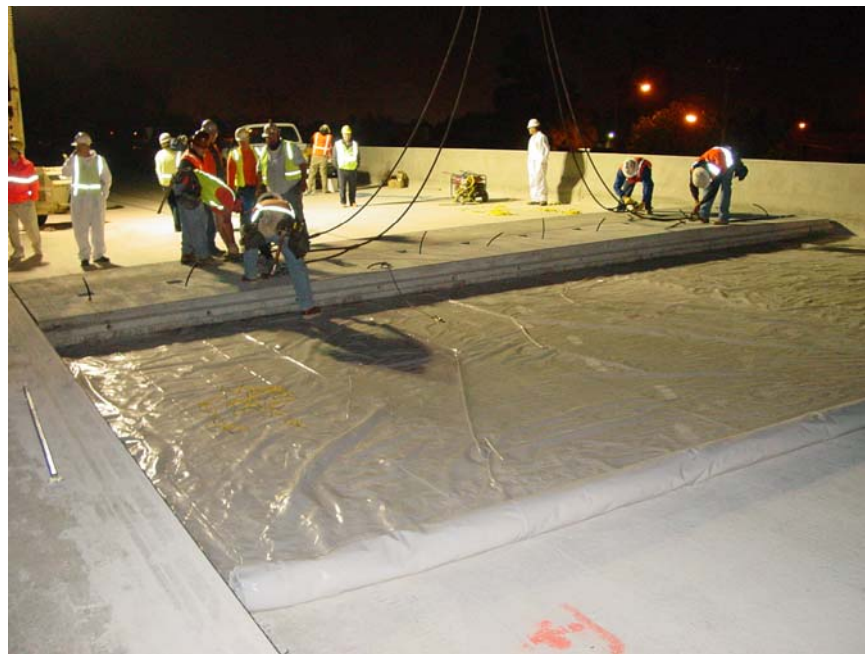
Figure 10. The polyethylene sheeting was rolled out just prior to the placement of each panel.
