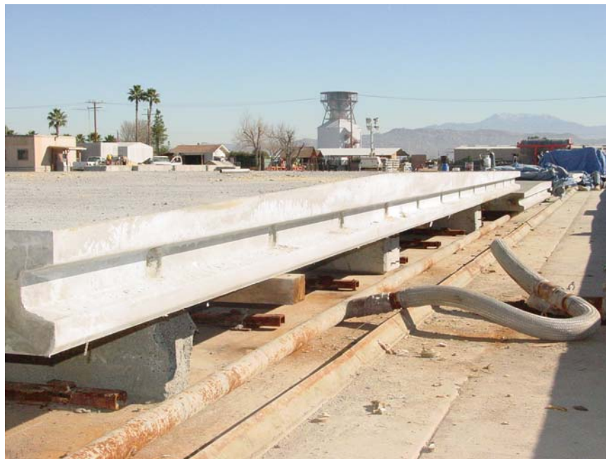
Figure 8. Typical precast panel after removal from the forms.
