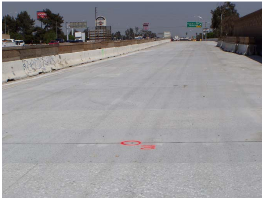
Figure 13. The finished precast pavement prior to opening to traffic.
