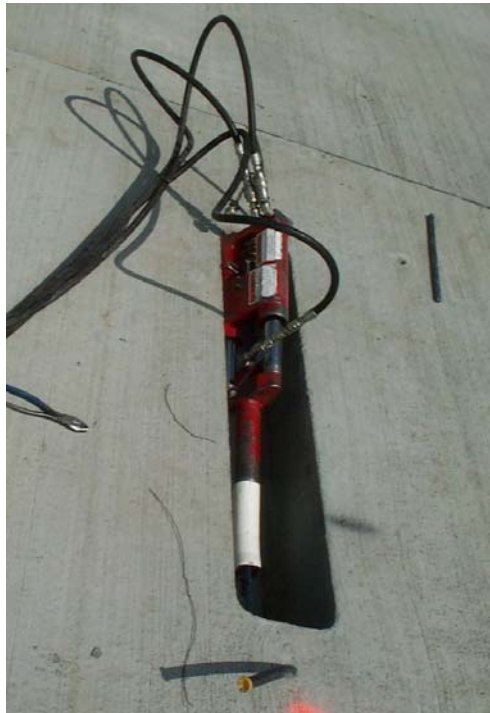
Figure 12. A monostrand stressing ram was used to tension the post-tensioning strands from the stressing pockets.
