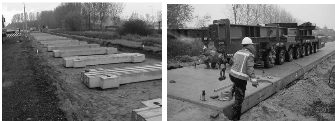
Figure 2. Installation (left) and leveling of the slabs (right) of the Modieslab test section along the motorway A50.
