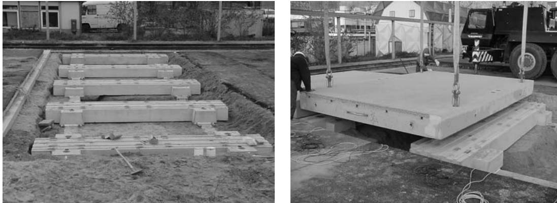
Figure 5. Construction of the original Modieslab test section.
