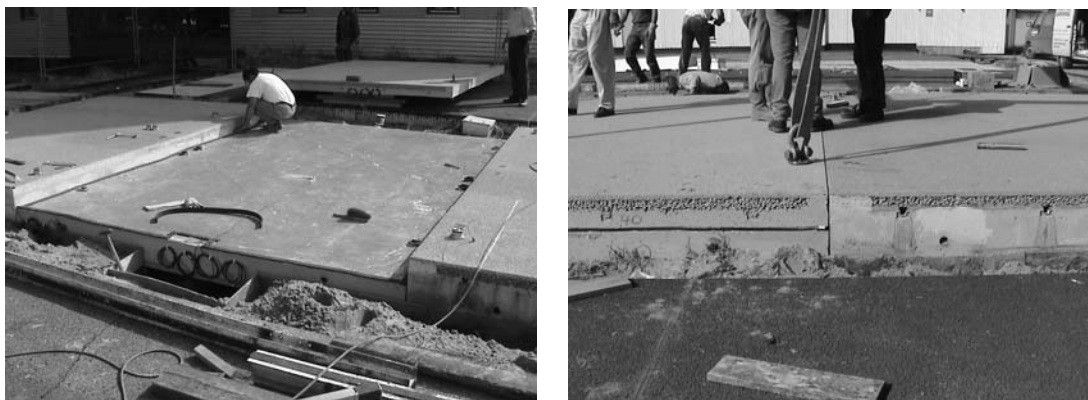
Figure 6. Installation of the two-layer slab 3 on the LINTRACK test section.
