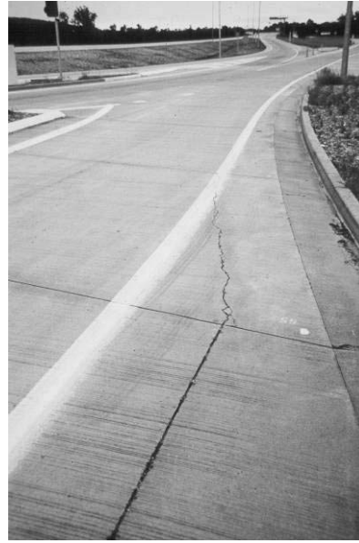
Figure 1.2: Jointing failure
