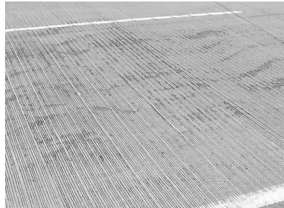
Figure 9.1. Close up of non-uniformity.
