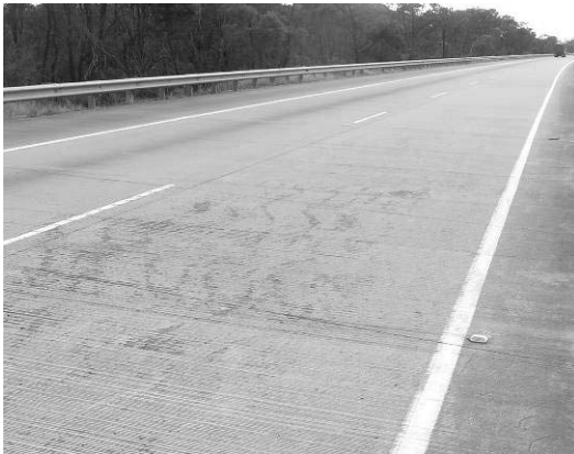
Figure 9.1. Non-uniform concrete
