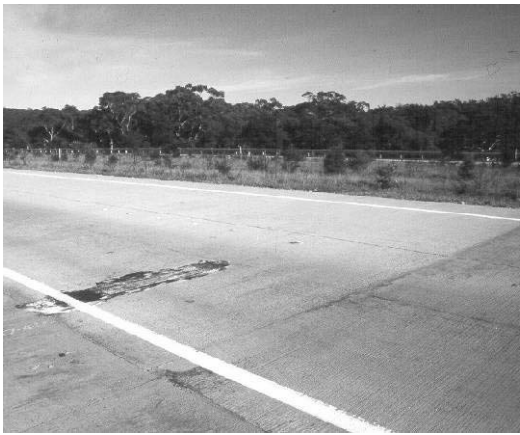
Figure 1.3: Compaction failure
