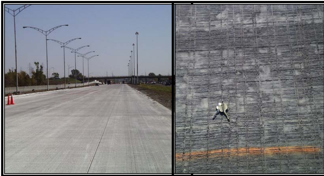
Figure 2 – Test section on Hwy 13 (Laval) and a view of the transverse tining
