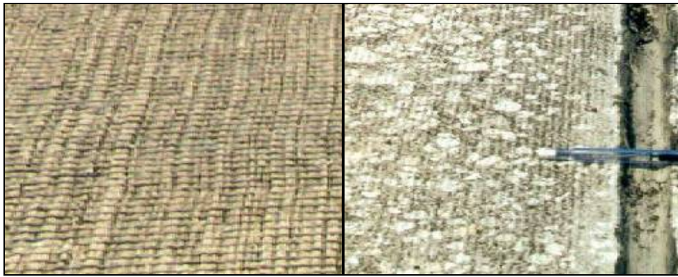
Figure 1. Original texture on runway (left), corduroy texture after milling (right).
