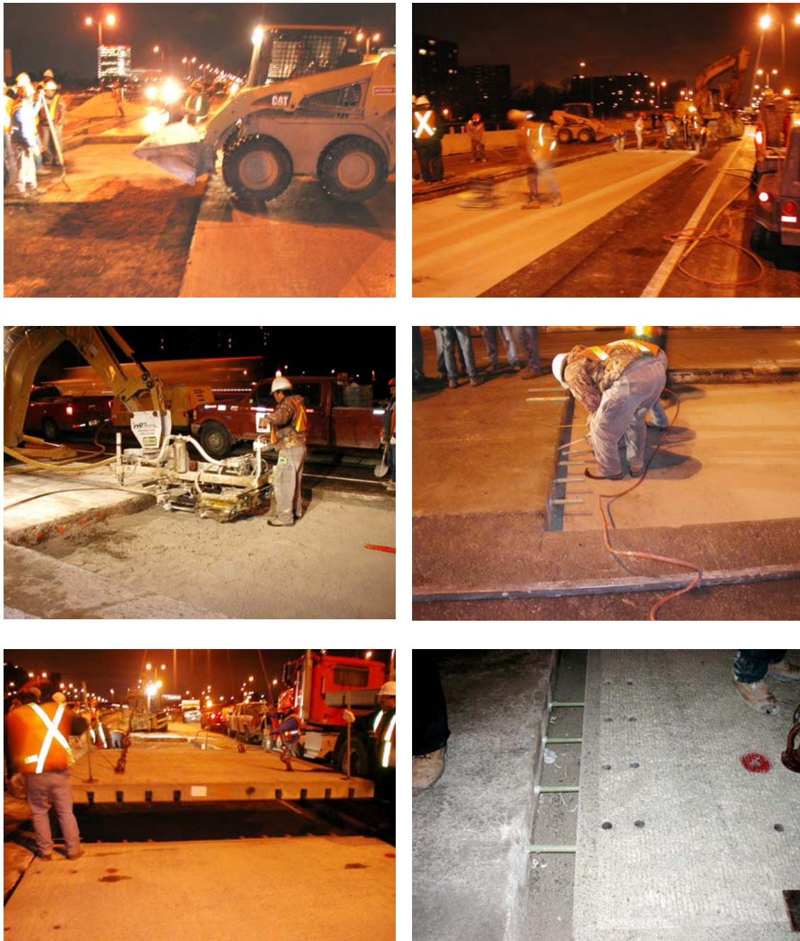
Figure 4. Construction sequence for Fort Miller Continuous pre-cast slab installation: a) placing crusher screenings into excavation with Bobcat, b) compacting crusher screenings using plate packer, c) gang-drilling dowel bar locations, d) fixing dowel bars with epoxy adhesive, e) lowering pre-cast slab, f) 180 mm gap between slab 6 and existing concrete.
