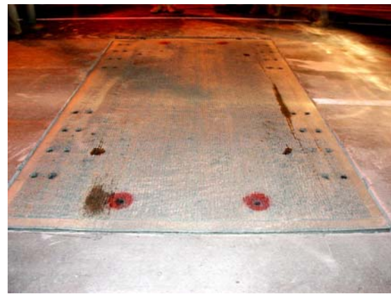
Figure 3. Construction sequence for Fort Miller Intermittent pre-cast slab installation: a) using full lane width leveling screed to fine grade crusher screenings, b) compacting crusher screenings using plate packer, c) dowel bars installed, ready to place pre-cast slab, d) lowering pre-cast slab, e) grout pump for grouting dowel bars, and f) final product, prior to grouting.
