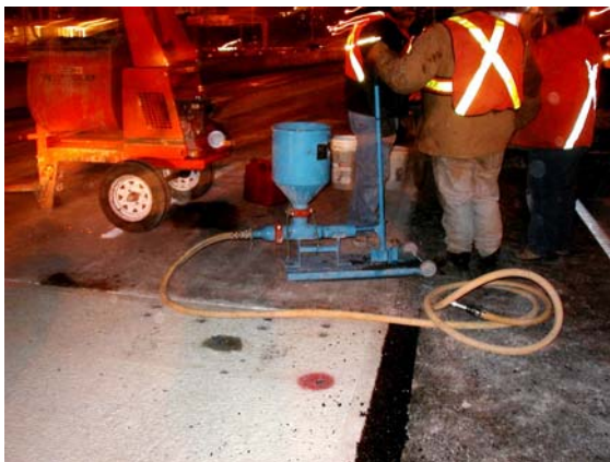
Figure 3. Construction sequence for Fort Miller Intermittent pre-cast slab installation: a) using full lane width leveling screed to fine grade crusher screenings, b) compacting crusher screenings using plate packer, c) dowel bars installed, ready to place pre-cast slab, d) lowering pre-cast slab, e) grout pump for grouting dowel bars, and f) final product, prior to grouting.
