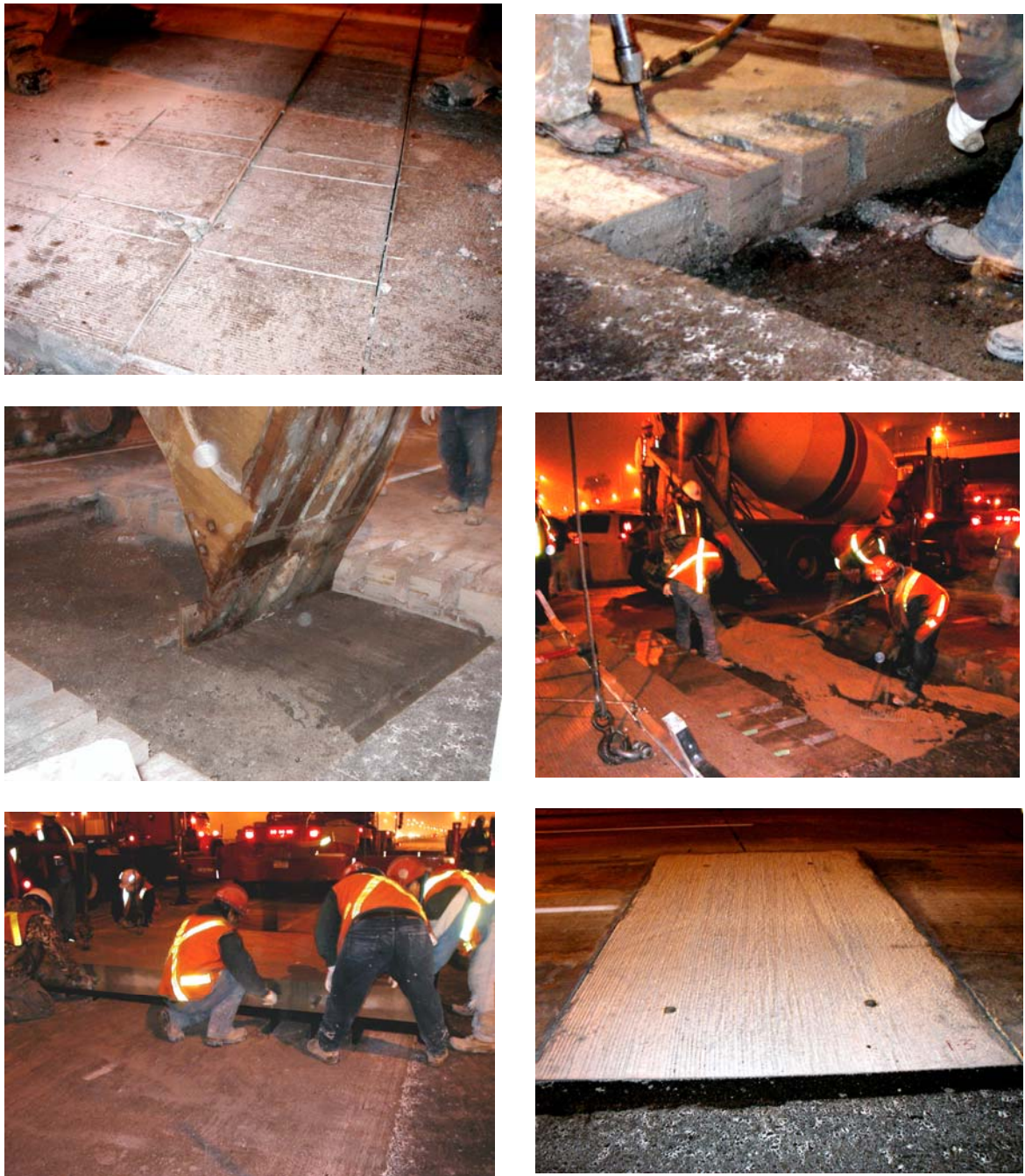
Figure 2. Construction sequence for Michigan Method pre-cast slab installation: a) perimeter sawcuts and sawcuts for dowel slots made the previous night, b) removal of dowel slots by jackhammer, c) scraping of CTB using a modified backhoe bucket, d) placement of flowable fill, e) lowering of pre-cast slab, and f) final product (slab 3).
