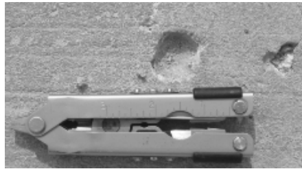
Figure 1. Example of severe popouts, Middle East Airbase
