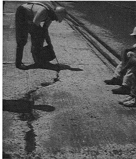
FIGURE 7 Application of monomer.
