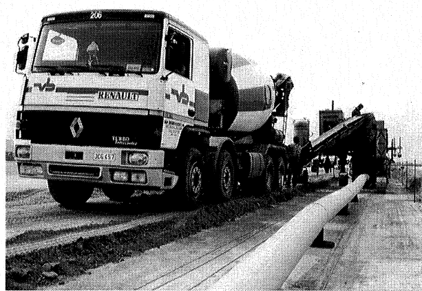
Figure 16. General view of the slotted drain construction
