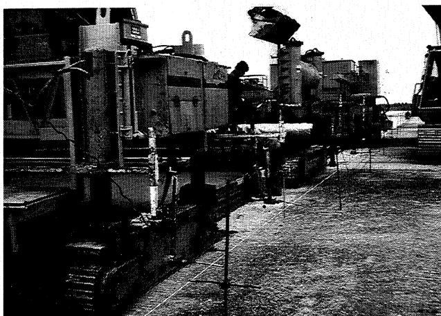
Figure 11. Construction of a 35 cm thick concrete pavement using two slipform pavers
