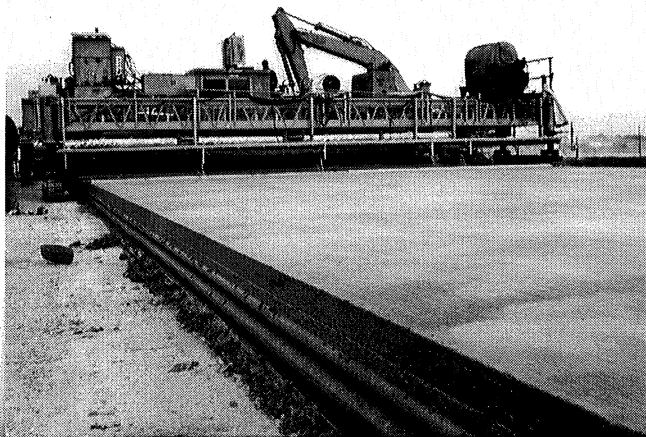
Figure 15. Brushed longitudinal grooves and perfect longitudinal construction joint
