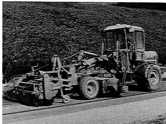
Figure 5 : Thorough brushing to remove the unhardened mortar the day after concreting.
