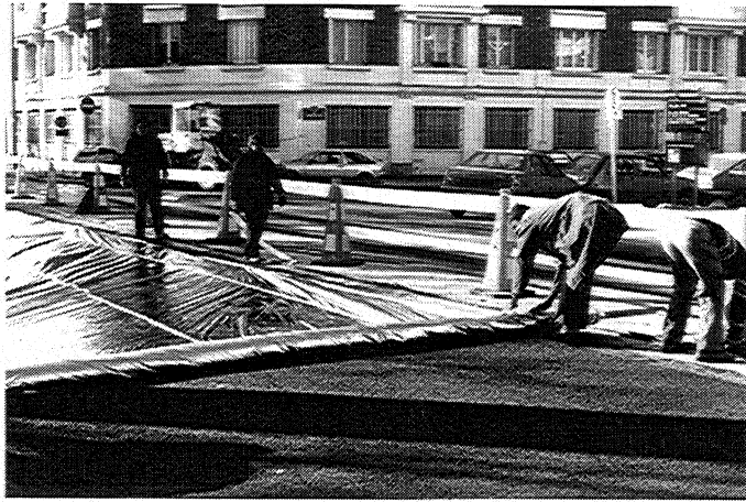
7 - A. Protection of fresh concrete with metallized polyethylene sheet: one of the key points for proper bonding, eliminating the temperature gradient.
