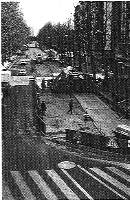
Figure 14: After excavation, placement of base concrete with slipform paver.
