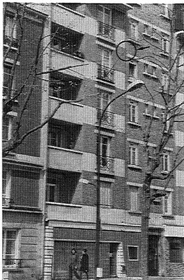
Figure 20: Positioning of measurement point for measuring the Leq 8h 20h. Acoustic measurements on building facades
