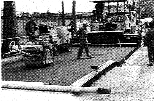
Figure 17: Modification of equipment, using a lighter compactor.
