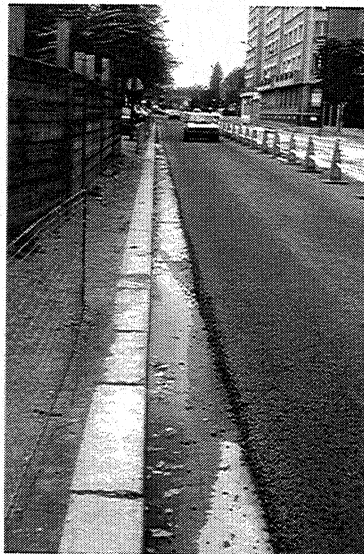
7 - C. Porous cement concrete pavement; general view.
