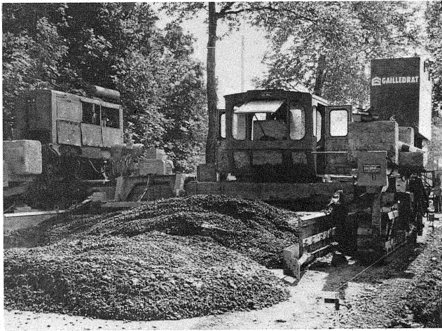
Fig. 3 Slip form on the County Road (C.D.) 940 jobsite (1974)
