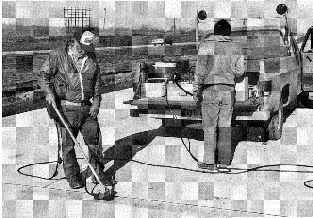
FIGURE 2 Radar Pass at Transverse Joint
