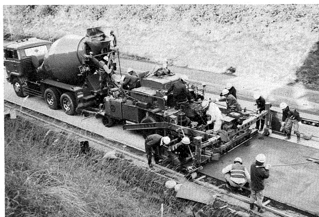
Photo 3 Concrete placing by using a paver
