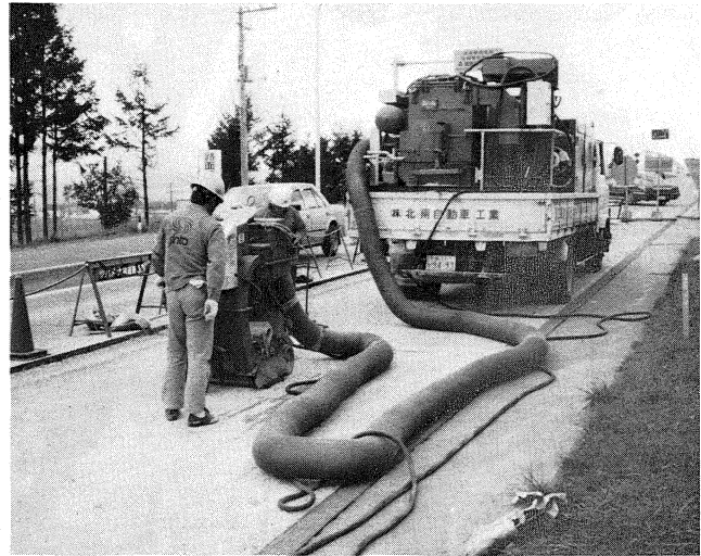
Photo 2 Shot blasting with \phi 1.4 mm steel balls
