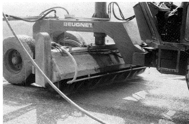
Fig 13. Stripping - Brooming of pavement
