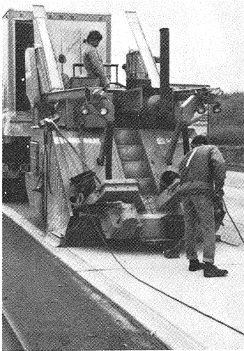
Figure 12 : Peening plant re-treating the surface of freeway A6-Essonne; maximum application with 2.25 m; execution speed: 1 to 15 m/minute.
